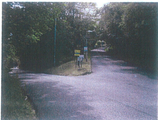
C282 (b) runs along Argyll Road shown on the right
